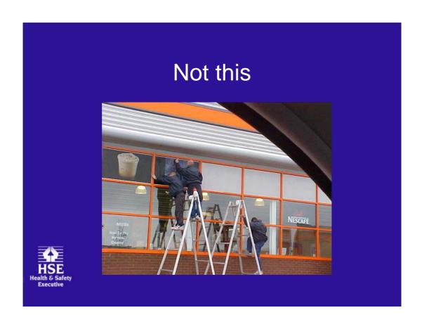
Tower would provide better ergonomic conditions ie sufficient space and dimensions, no overreaching or overbalancing etc
